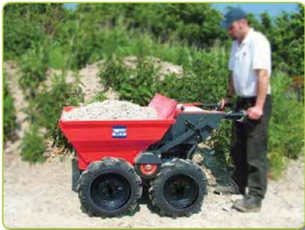
Site Operator Using the HTL350 for Fast and Easy Transportation of Gravel
