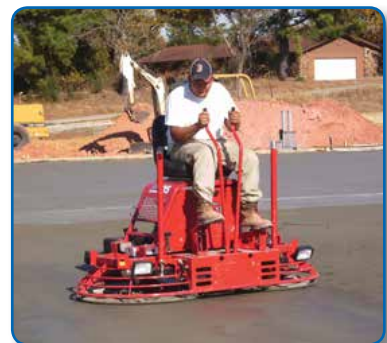
Operator at Work with the Ride-On Trowel
