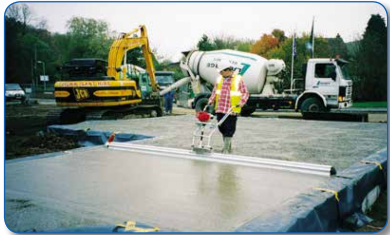
Operator at Work with the HOPPT® DUOSCREED
